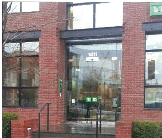
Multi-paned STOREFRONT windows and glass doors
