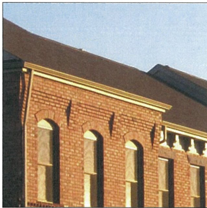
Pitched roof with projecting CORNICE
