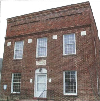
Brick building walls
