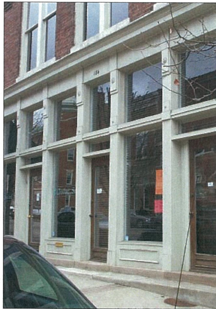
Cast iron STOREFRONT with brick second STORY
