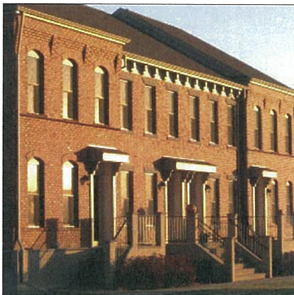
Newly constructed brick townhouses with architectural detailing
