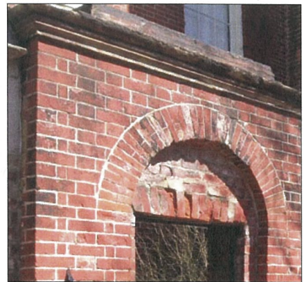
Parapet wall with COPING
