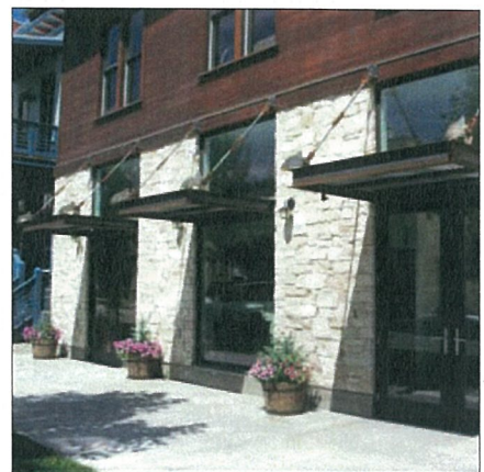
Building FACADES with limestone ground floor and wood siding above.
