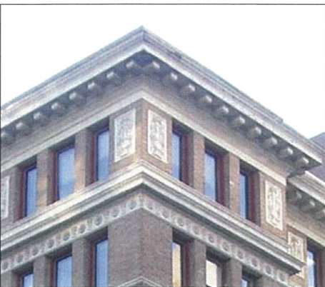
Parapet wall with projecting CORNICE
