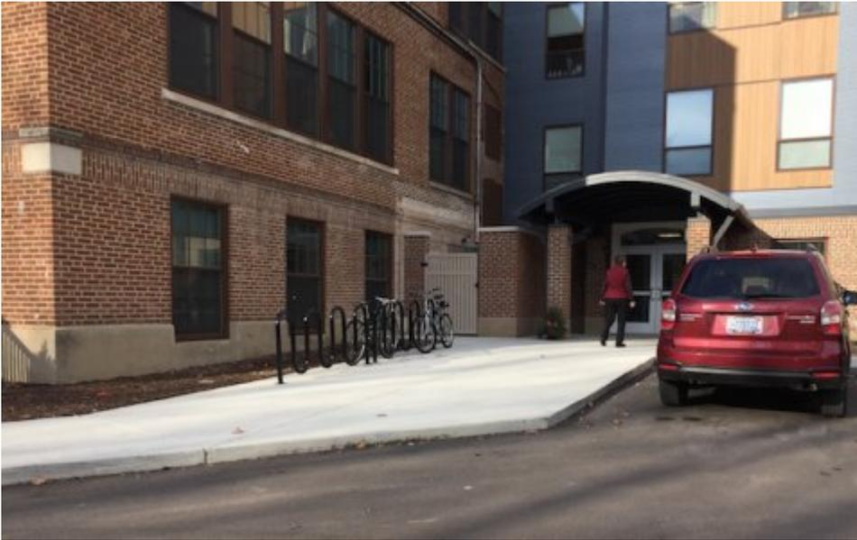
There is no ramp or curb-cut near the front door of the residences (above). Instead, the cut providing a ramp from the walkway level to the parking lot level is halfway-down the parking lot space, and was built in such a way that water pools at the base of the small ramp.
