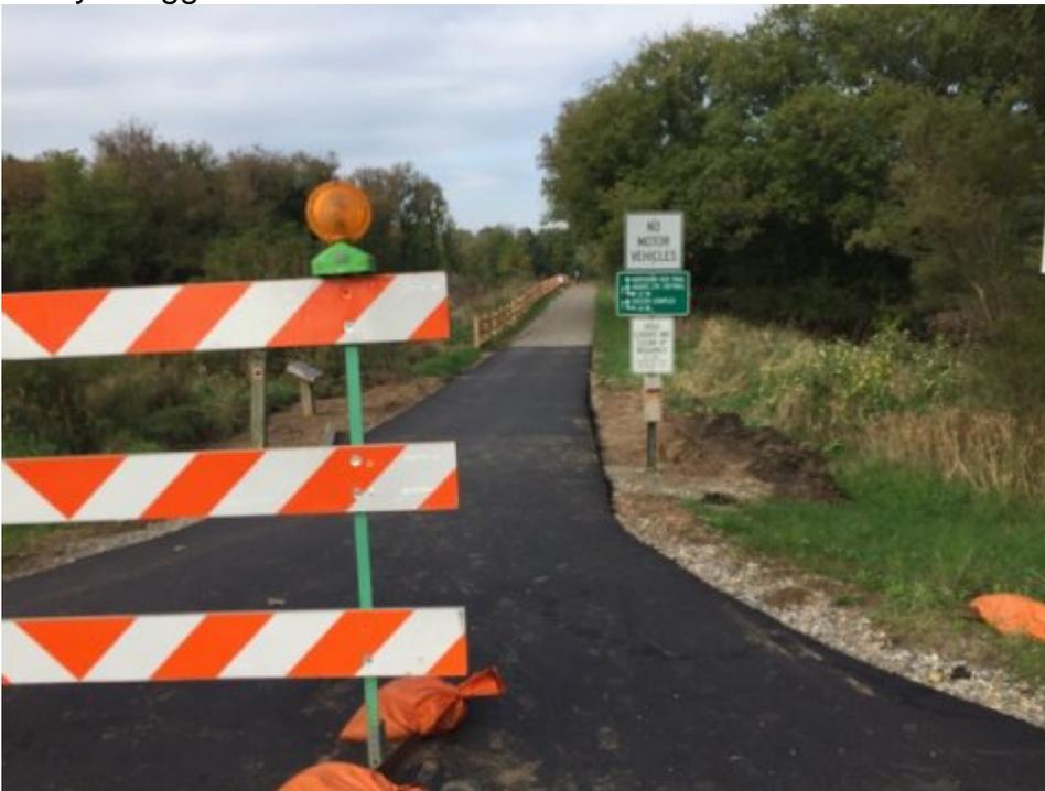
Workers were able to complete all of the planned asphalt improvements to East Lansing's Northern Tier Trail system before the winter weather hit, including fixing a dramatic drop-off where the trail meets the sidewalk of Abbot Road near the East Lansing Fire Department (shown above).
